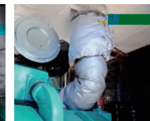
Built-in high-temperature protective material
